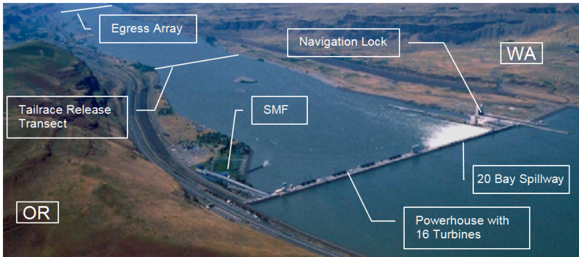
Figure 1.2. Aerial View of John Day Dam. SMF = Smolt Monitoring Facility.
